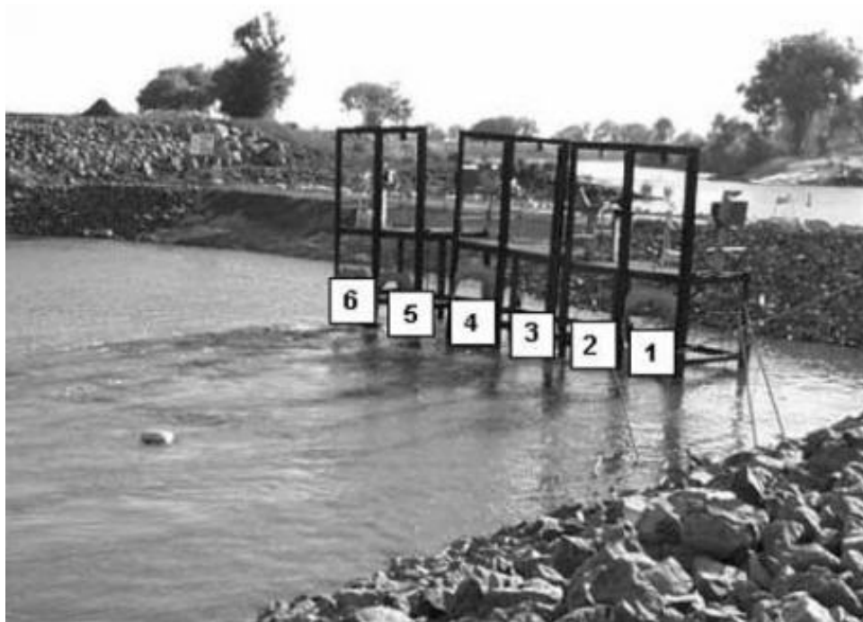
Figure 3.12-1 Photograph of Head of Old River Barrier (top) from DWR TBP (2008); photograph showing location and numbering of six culverts through the 2002 Head of Old River Barrier (bottom) from DWR (2003).
