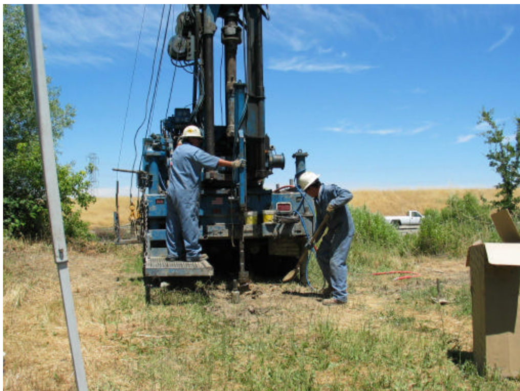
Figure 9. Auger drilling on the west bank of Weir No. 2
