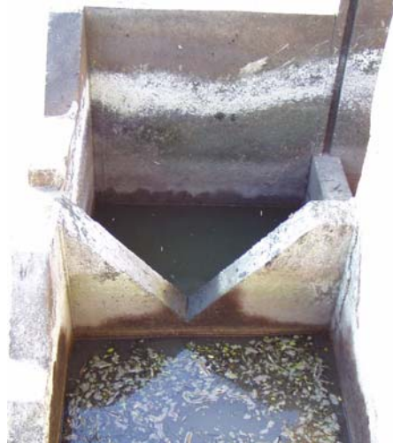
Figure 5. V-notch of the existing pool and weir fish ladder
