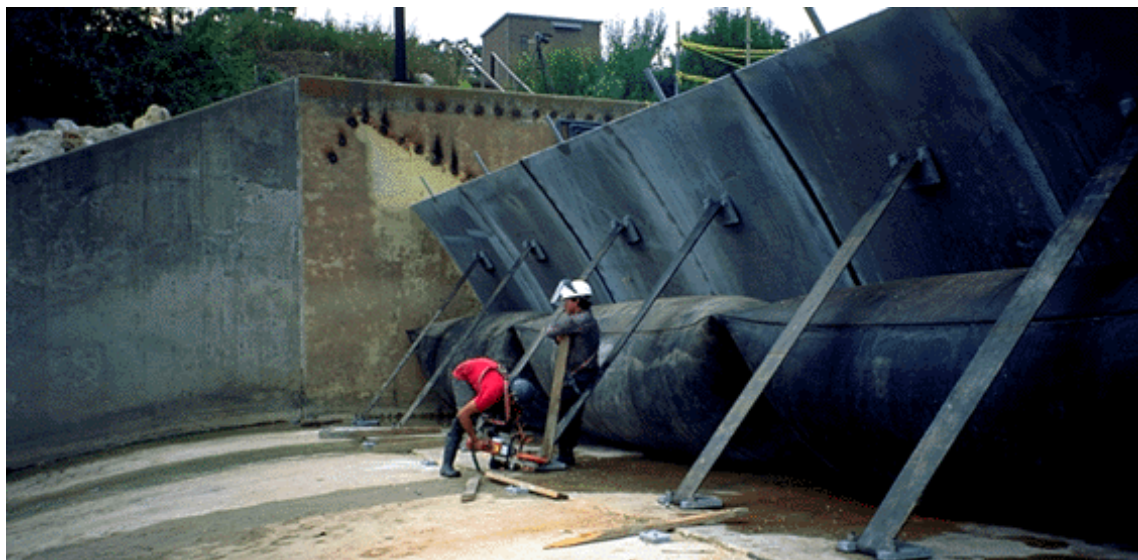
Figure 13. Installation of spillway gates
