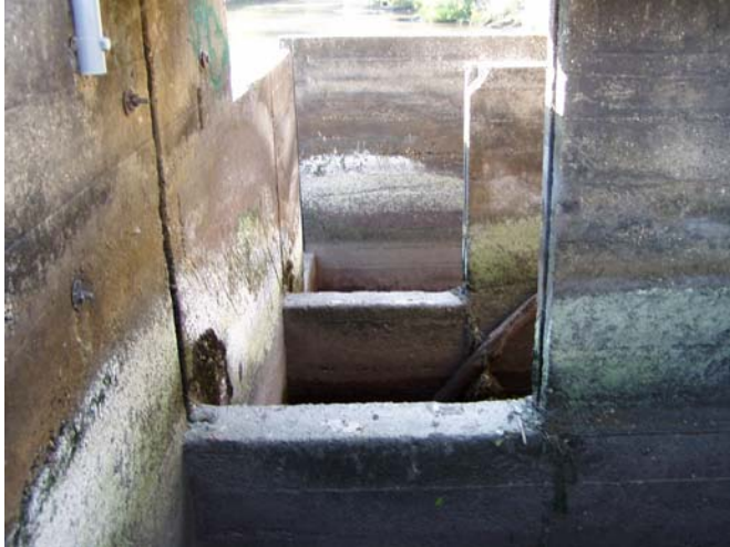
Figure 4. Rectangular weir of the existing pool and weir fish ladder
