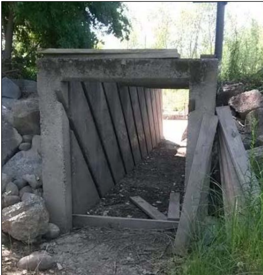
Figure 1-2 View of Existing Modified Denil-type Fish Ladder with Stoplogs and Interior Baffles Removed, Looking Downstream
